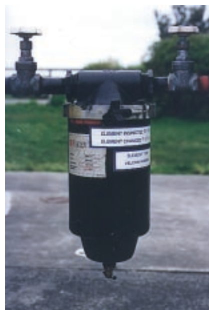
Ensure that your aircraft refuelling system has the approved fuel filters fitted so that the chances of static build-up are reduced.
