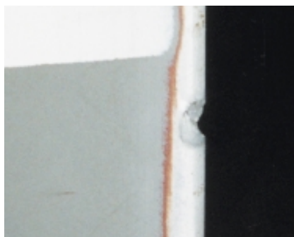
Stone-chip damage such as this should be referred to a LAME immediately.
