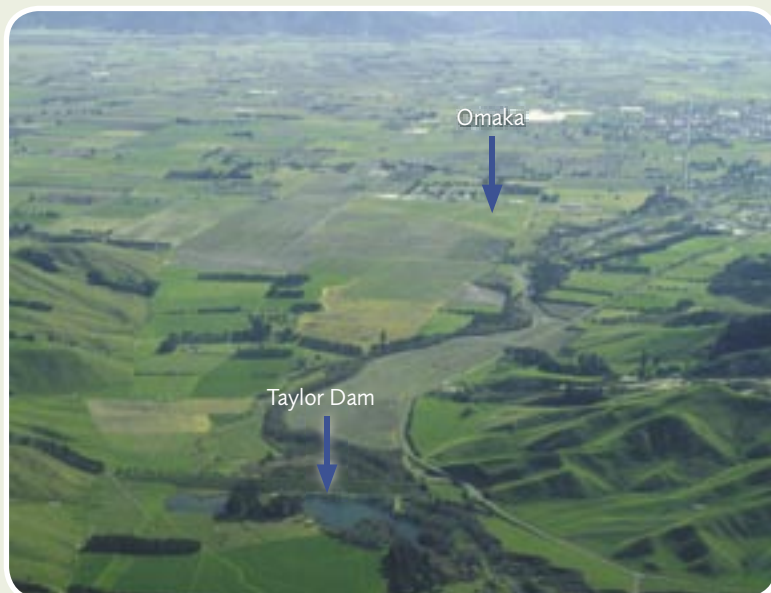
Taylor Dam looking north towards Omaka aerodrome.
