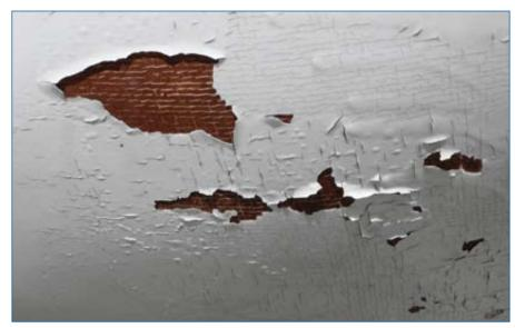
Poor preparation and painting caused this blistering.
