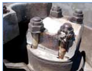
The fracture surface of the failed leg. The fatigue portion of the crack is the rust-coloured area.
