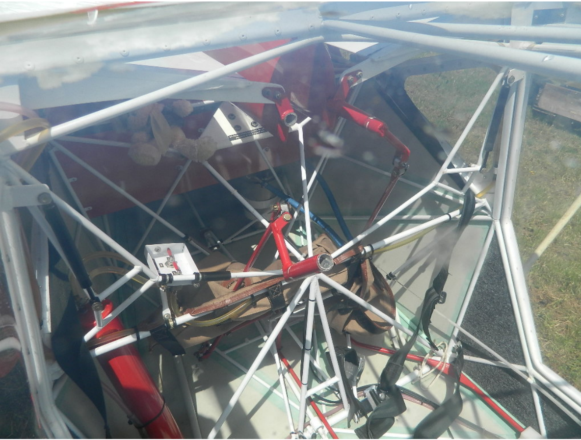
Photograph 1 – Starboard flaperon aluminium spar tube failure at the joint where this tube enters the 4130 steel bellcrank (Note: In these photographs the aircraft wings are folded).
