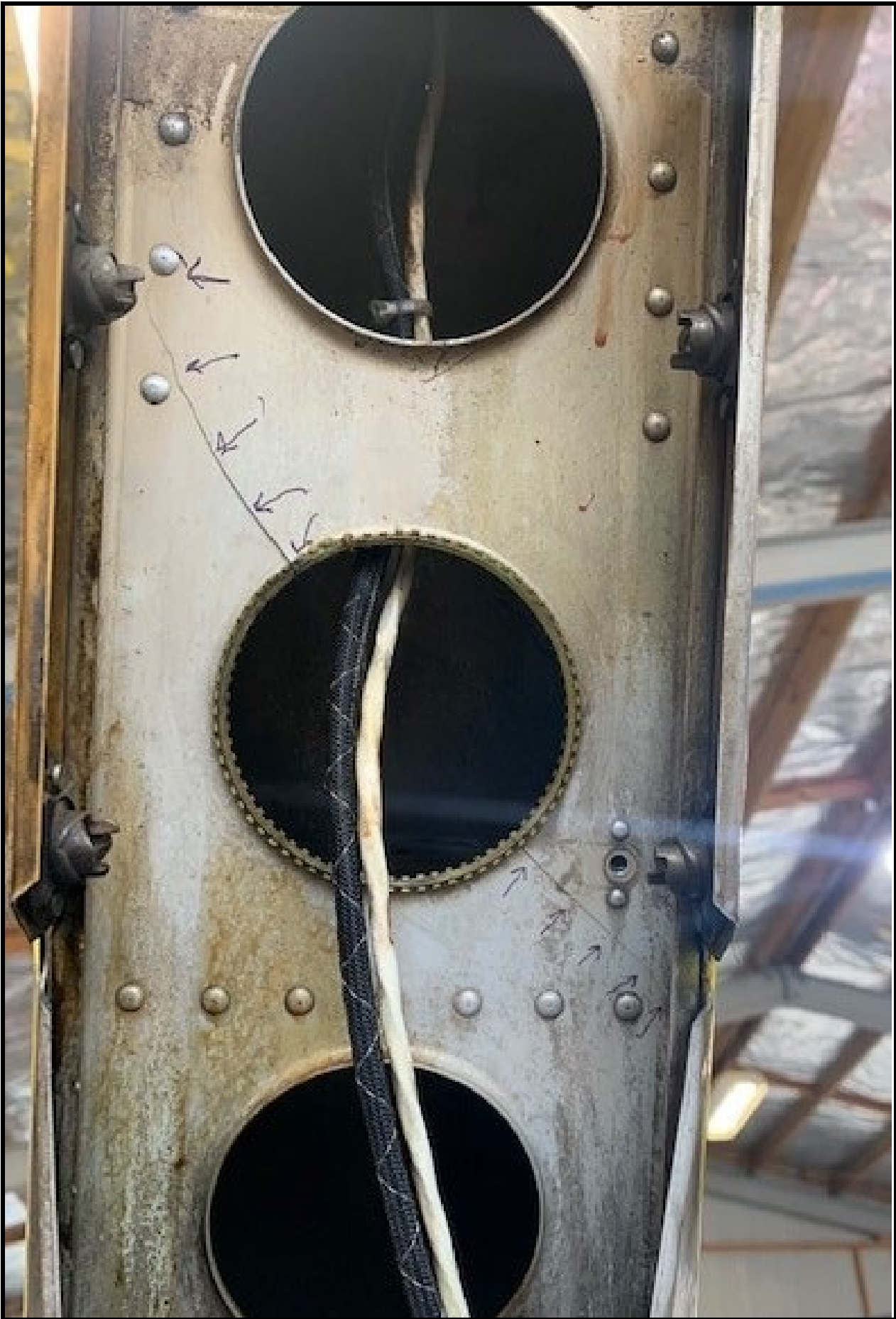
Photo 2: Location of cracks found in vertical fin spar with actuator removed.
